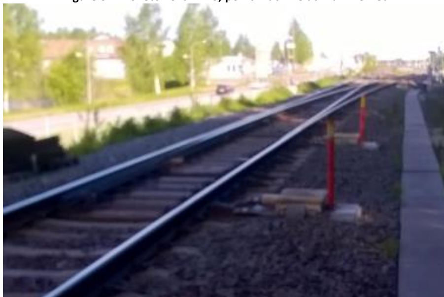
Figure 3.12: Switch with 2 point machine in switch panel and two point machines in crossing panel
