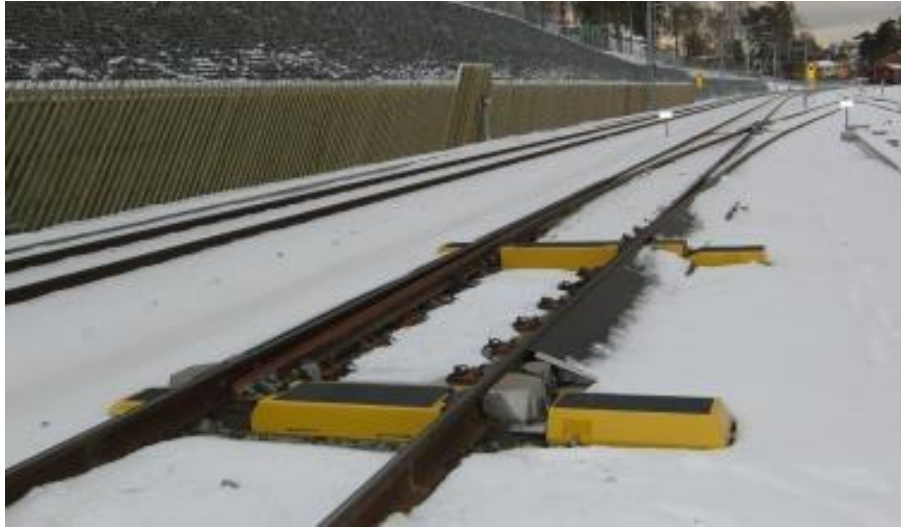
Figure 3.14: Switch with 2 hydraulic-electric point machine in switch panel
