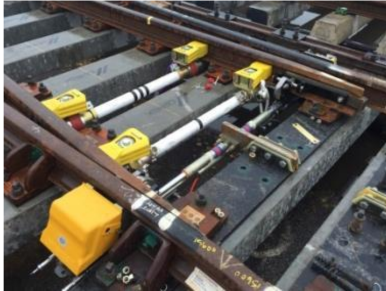
Figure 3.1: Rail Point Clamp Lock photograph
