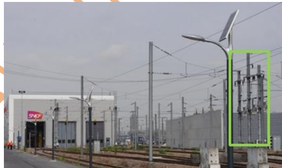
Figure 2.5 : SNCF Railway maintenance centre, powered by catenaries
